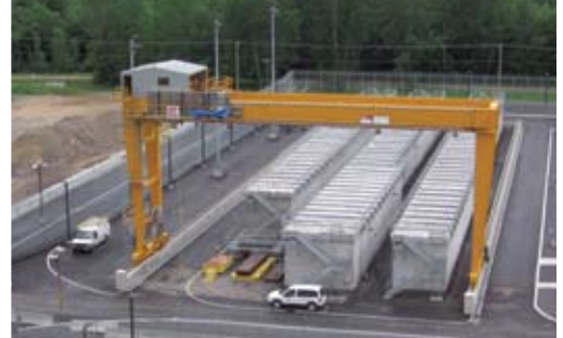
Phase 1 of the Gentilly-2 SRWMF, constructed in 2007 and 2008
