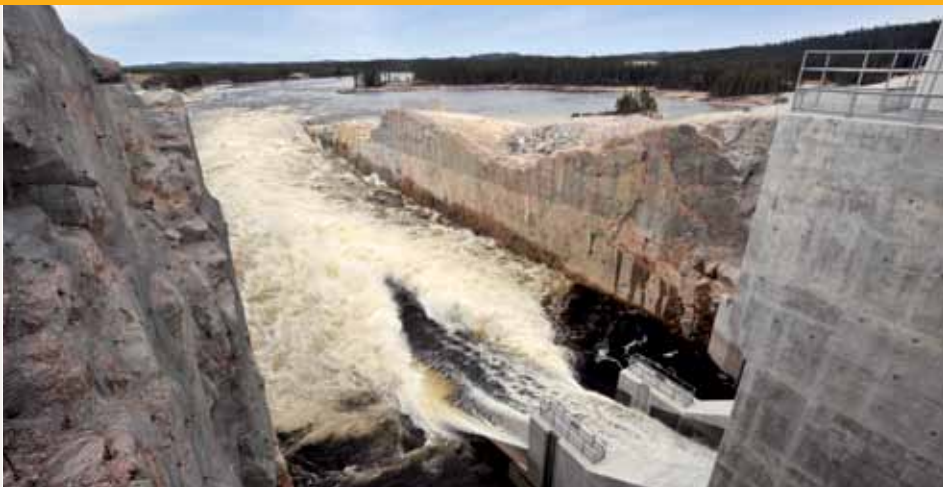
The Rupert Spillway
