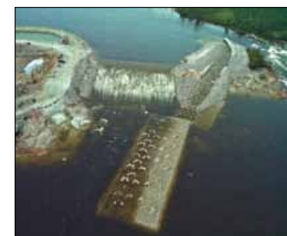
Weir at KP 290. To the right of the weir is the fish pass, a small channel allowing the free movement of fish, which swim up past the weir. A spawning ground for sturgeon has been developed downstream of the
