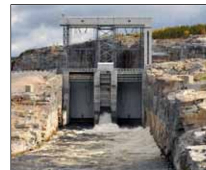
Rupert spillway has three gates. Instream flow is released through the middle one.
