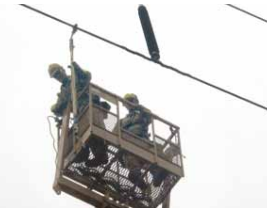
Installing an interphase spacer
