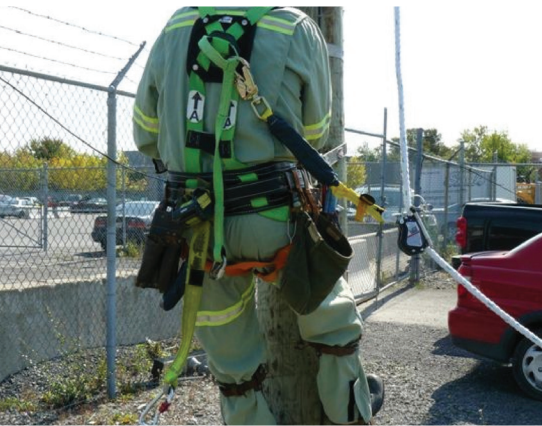
Using a vertical lifeline to climb a wood pole
