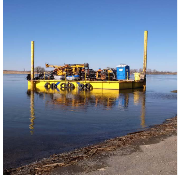
Barge used for drilling
