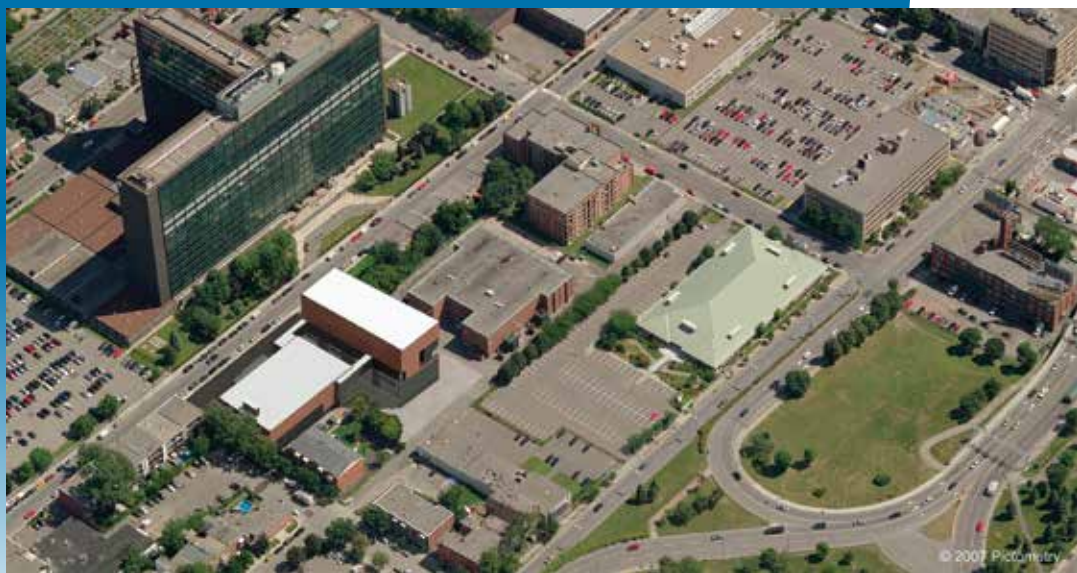
Planned substation (simulation)
