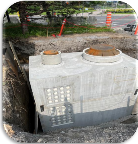
Construction of ducts and underground chambers
