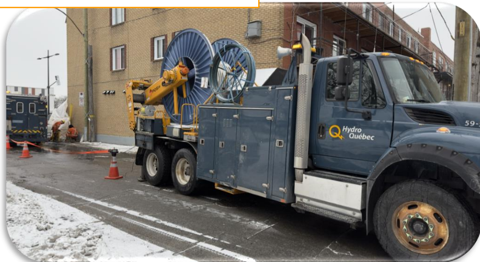
Underground cable installation
