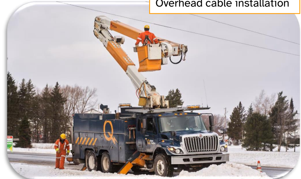
Overhead cable installation
