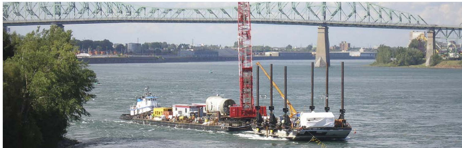
The RER Hydro turbine had a planned capacity of 100 kW.
