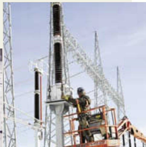
Construction of Outaouais substation.
