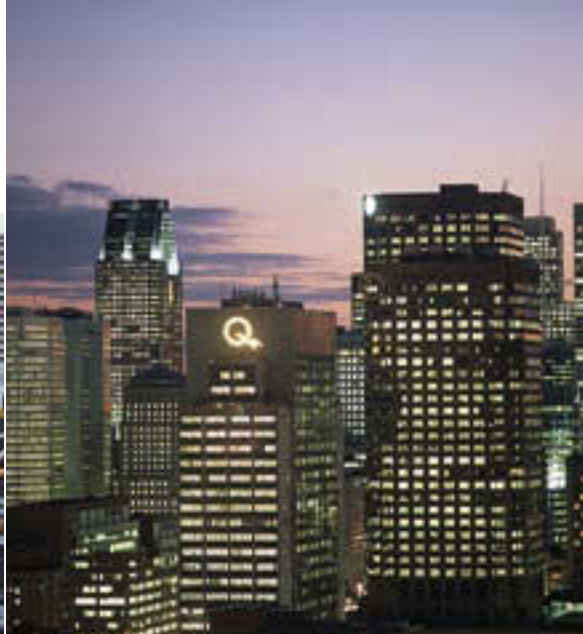
The sign on top of the head office building has gone "green". A new device to regulate on/off cycles and the use of T-8 lamps will save 43,000 kWh annually.
