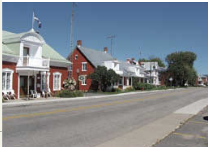
Distribution system undergrounding in Yamachiche has improved the landscape.
