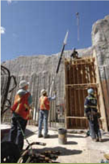
Working on the Rupert spillway.
