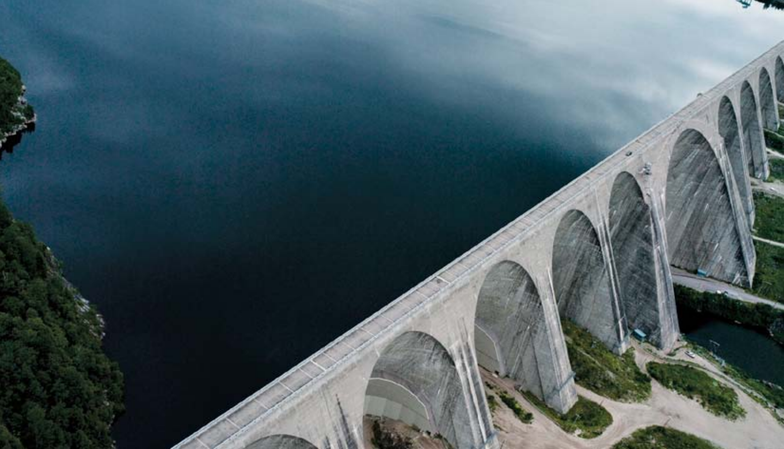
Daniel-Johnson dam, built in 1968, is the world's largest multiple-arch dam.
