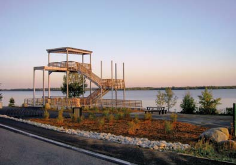
Lookout built with funding from Hydro-Québec by the regional county municipality of Argenteuil on the site of Carillon generating station in the Outaouais region.
