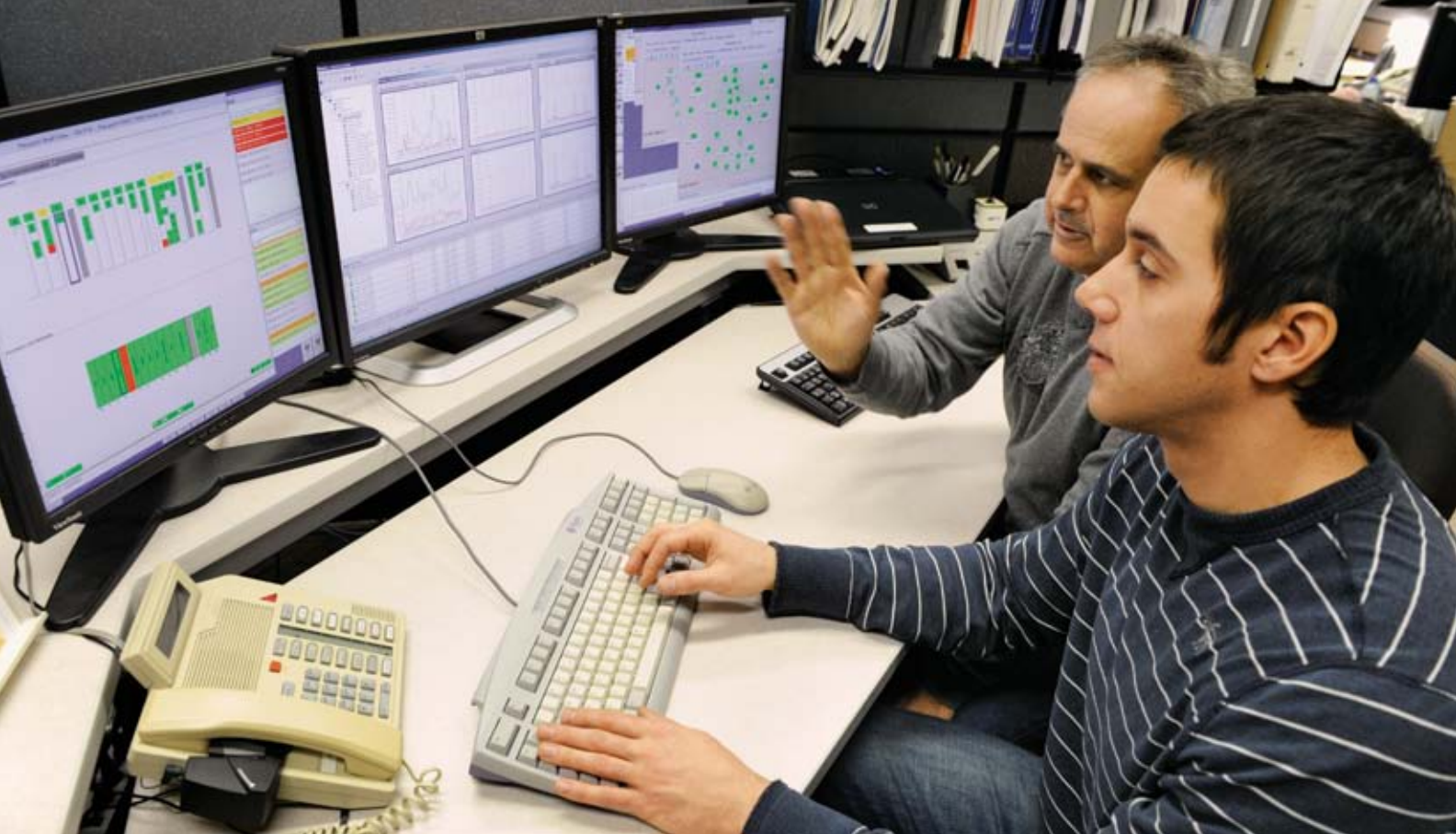
Technicians Carl Cyr and Robert Dubois work side by side in the telecommunications control centre. The objective is knowledge transfer.
