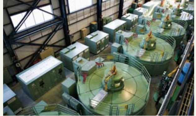
Rapides-des-Coeurs generating station.
