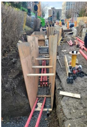
Rebuilding the underground power system.
