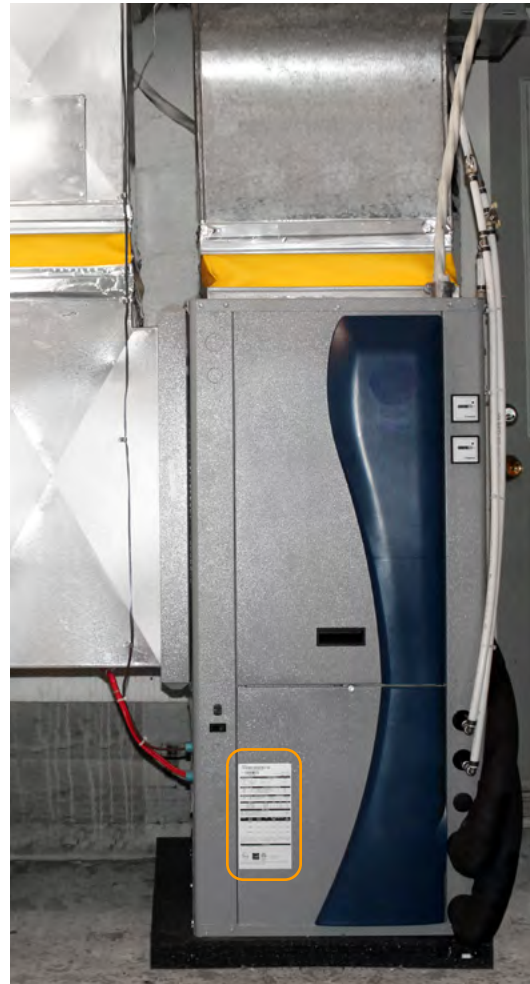
Location of the label on an indoor unit of a central, air-to-air split-system heat pump.
